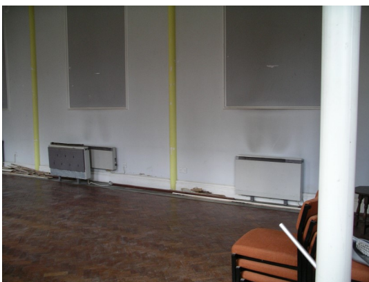
Milner Hall before refurbishment
